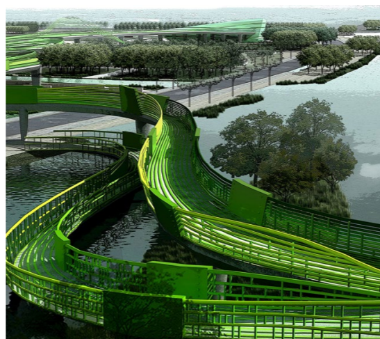
CHINE – Suining Sleeve bridge
