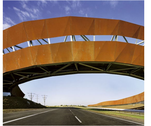
AUSTRALIE – Craigieburn Bypass
