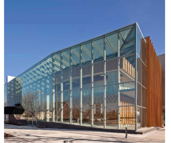
CANADA – Centre for Engineering Innovation
