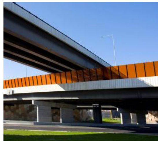
AUSTRALIE – Craigieburn Bypass
