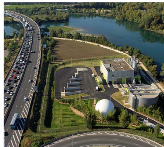
FRANCE – Lyon – Station d'Épuration
