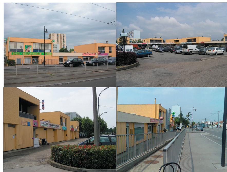
Centre commercial Palmer
