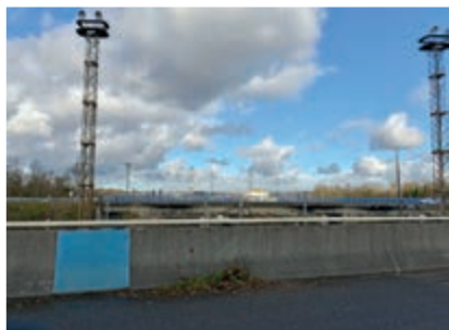
Grands mâts SNCF - Villenave-d'Ornon
